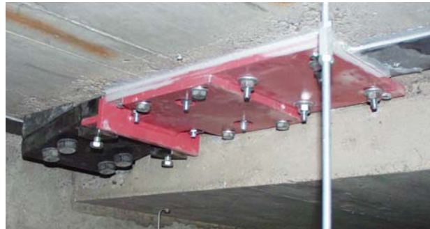
Fig. 5 Dead-end anchorage with temporary clamp.
