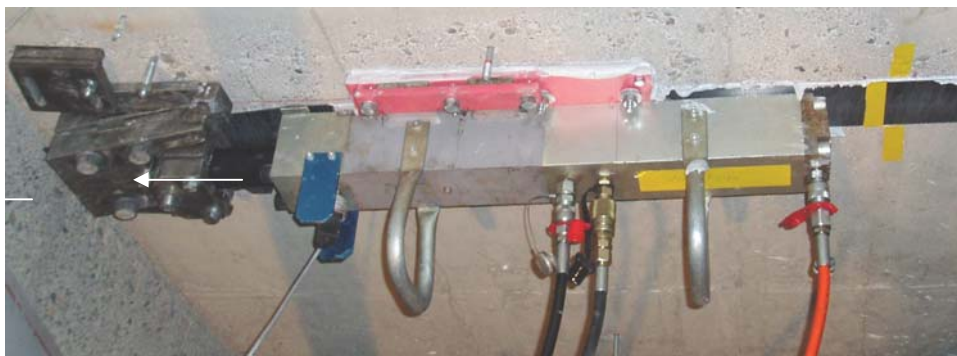
Fig. 4 Prestressing jack with temporary clamp, arrow indicates direction of prestressing.
